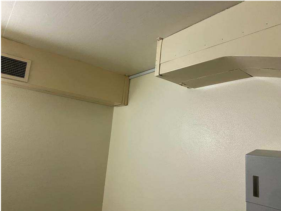
Image 2 : Ground Floor Parent Toilet Supply & Exhaust Ducts
