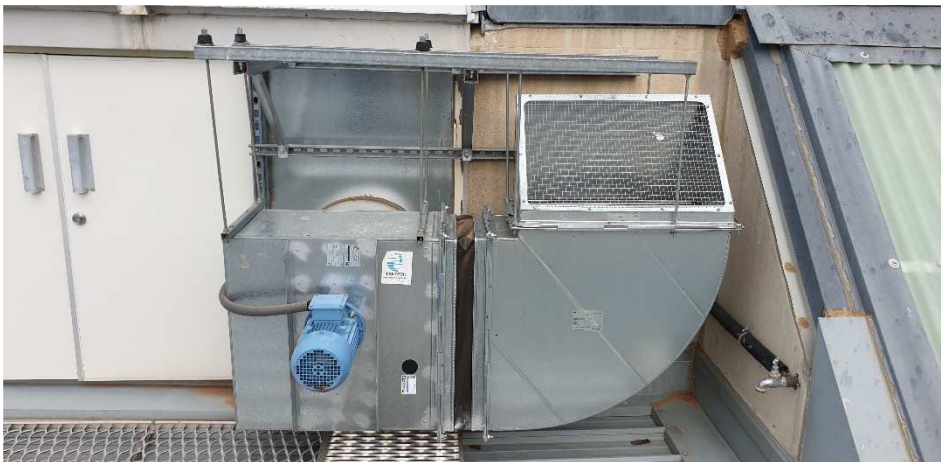
Image 4 : Centralised Exhaust Fans
