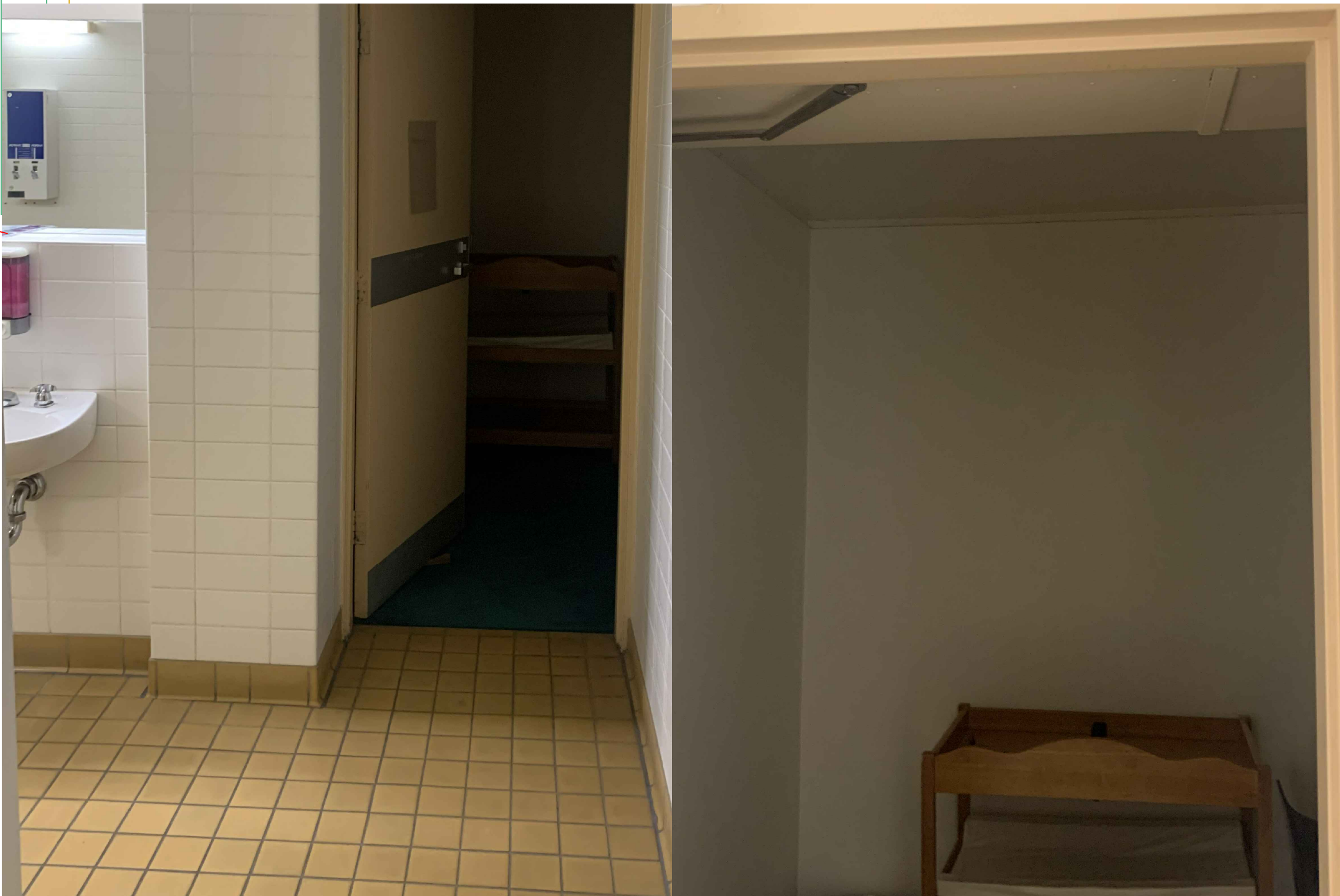
View looking towards entry door to the proposed accessible toilet. To the left is the existing ladies toilet. This entry door will be bricked up.
