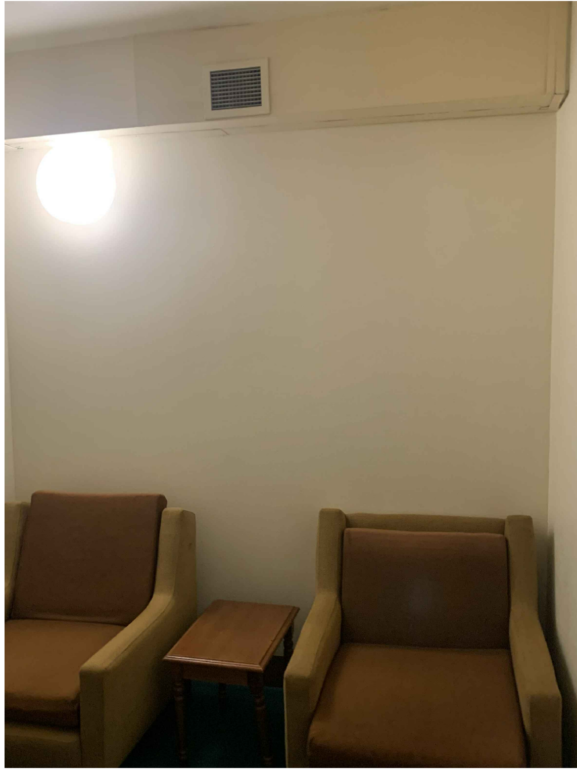
View looking towards far wall (north) of proposed accessible toilet. This wall needs to have the auto door installed. View shows the mechanical duct at the top that need to be removed.
