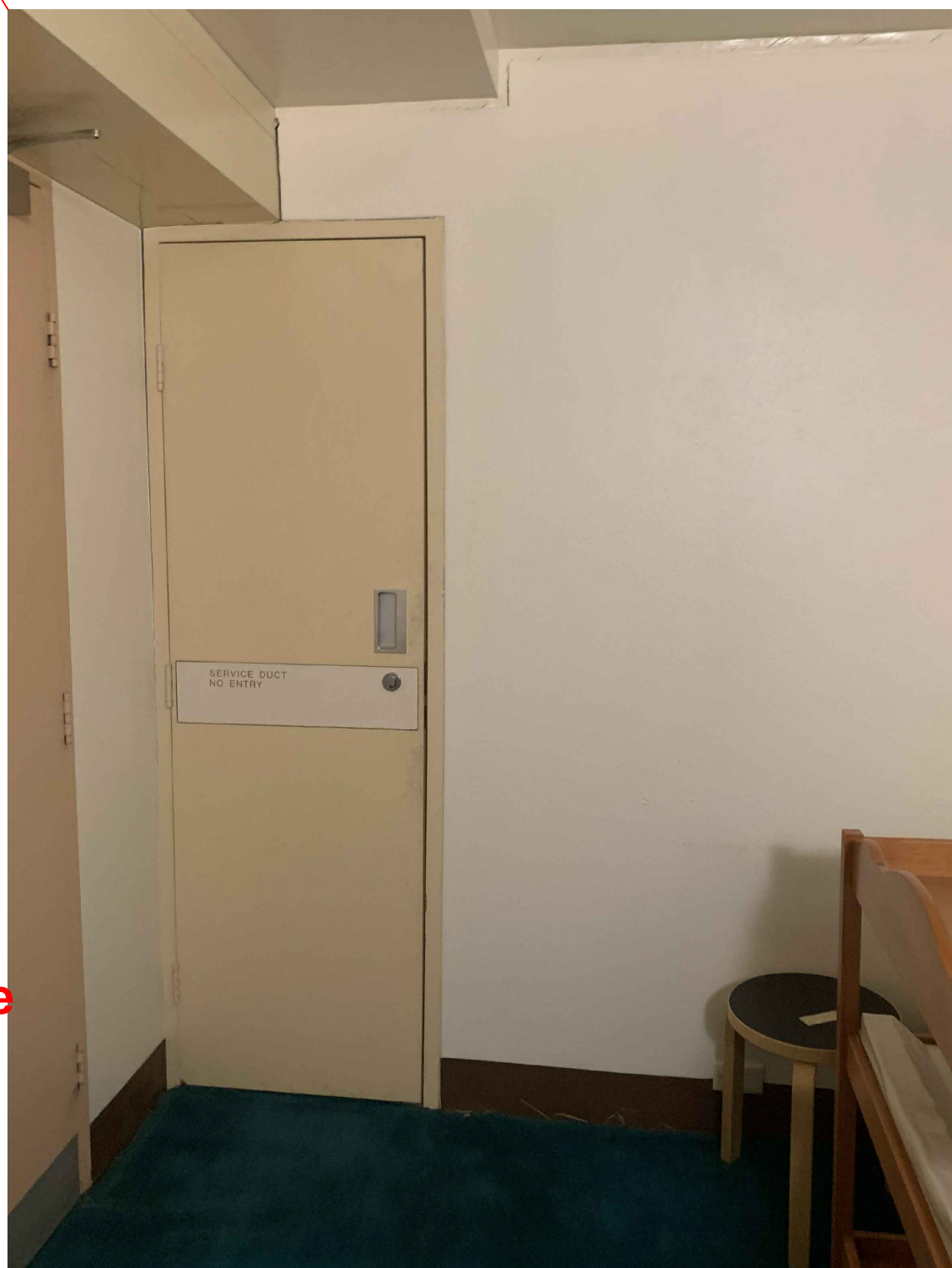
View looking towards near wall (south) of proposed accessible toilet. This wall has a access door to the services riser behind. View shows the mechanical duct at the top left that needs to be modified.
