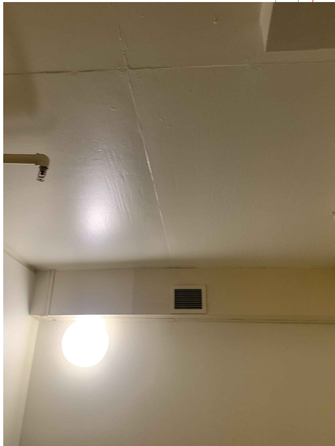
View looking towards upper far wall (north) of proposed accessible toilet. This wall needs to have the auto door installed. View shows the mechanical duct at the top that need to be removed. The view also shows the concrete ceiling.
